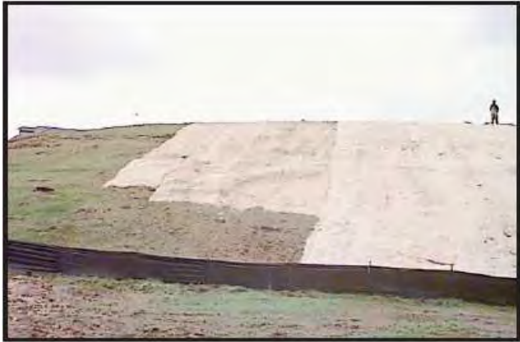
Figure 3 - Coconut matting and silt fence (Source: CIRIA, 2006 12 )
