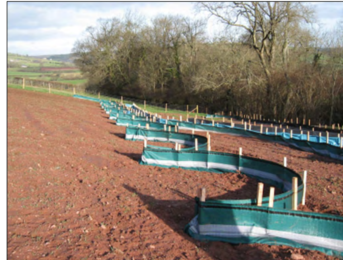
Figure 2 - Example of good practice in silt fence installation (Source: Geosynthetics, 2021 11 )
