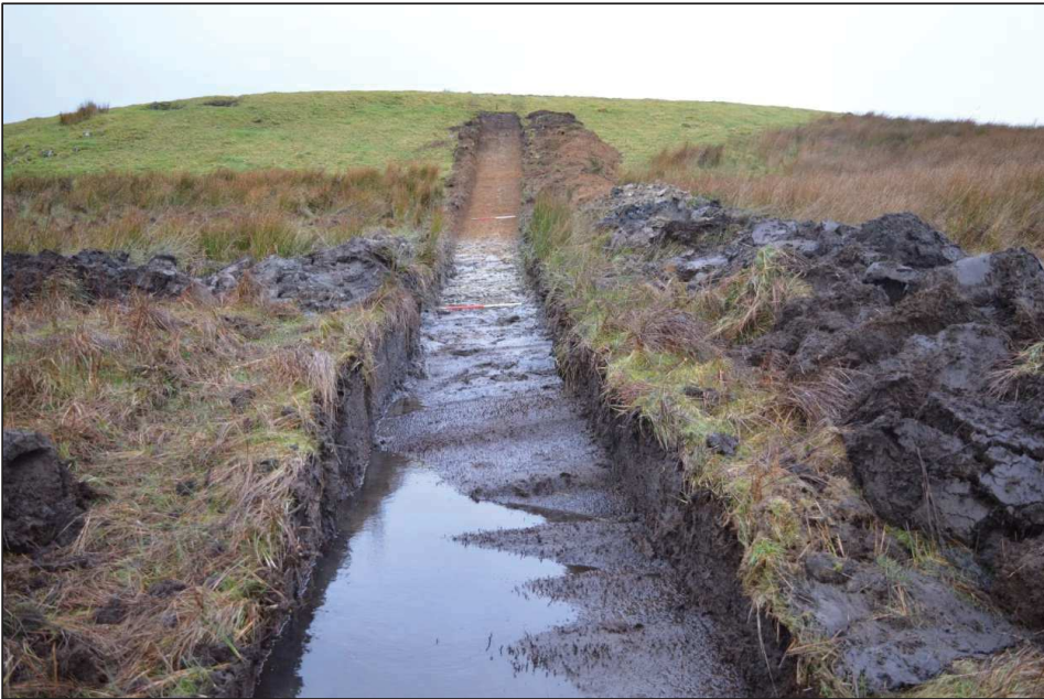
Fig. 17: Trench 7 from the south-east, showing the waterlogged ground. CPAT 4967-0042
