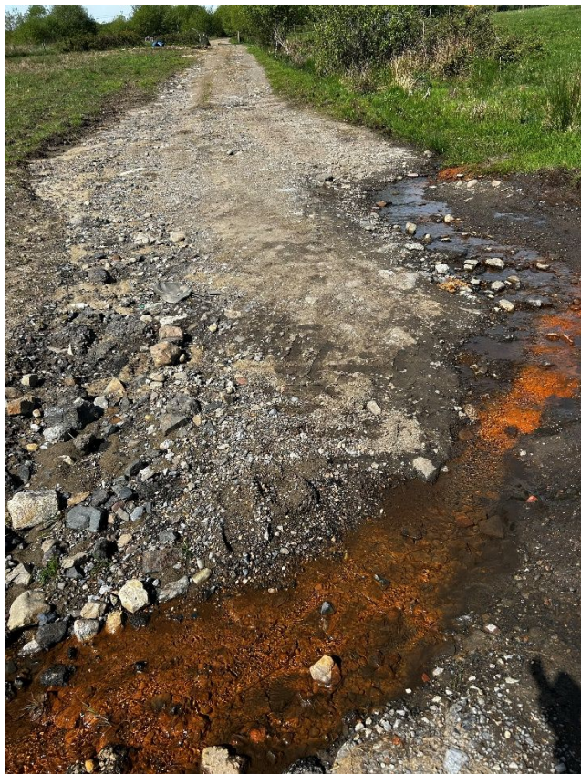
Fields in southern land parcel showing a small surface water flow path across the gravel track with ocherous staining
