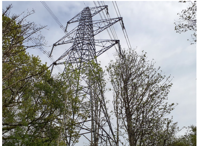
View looking north-east at edge of woodland
